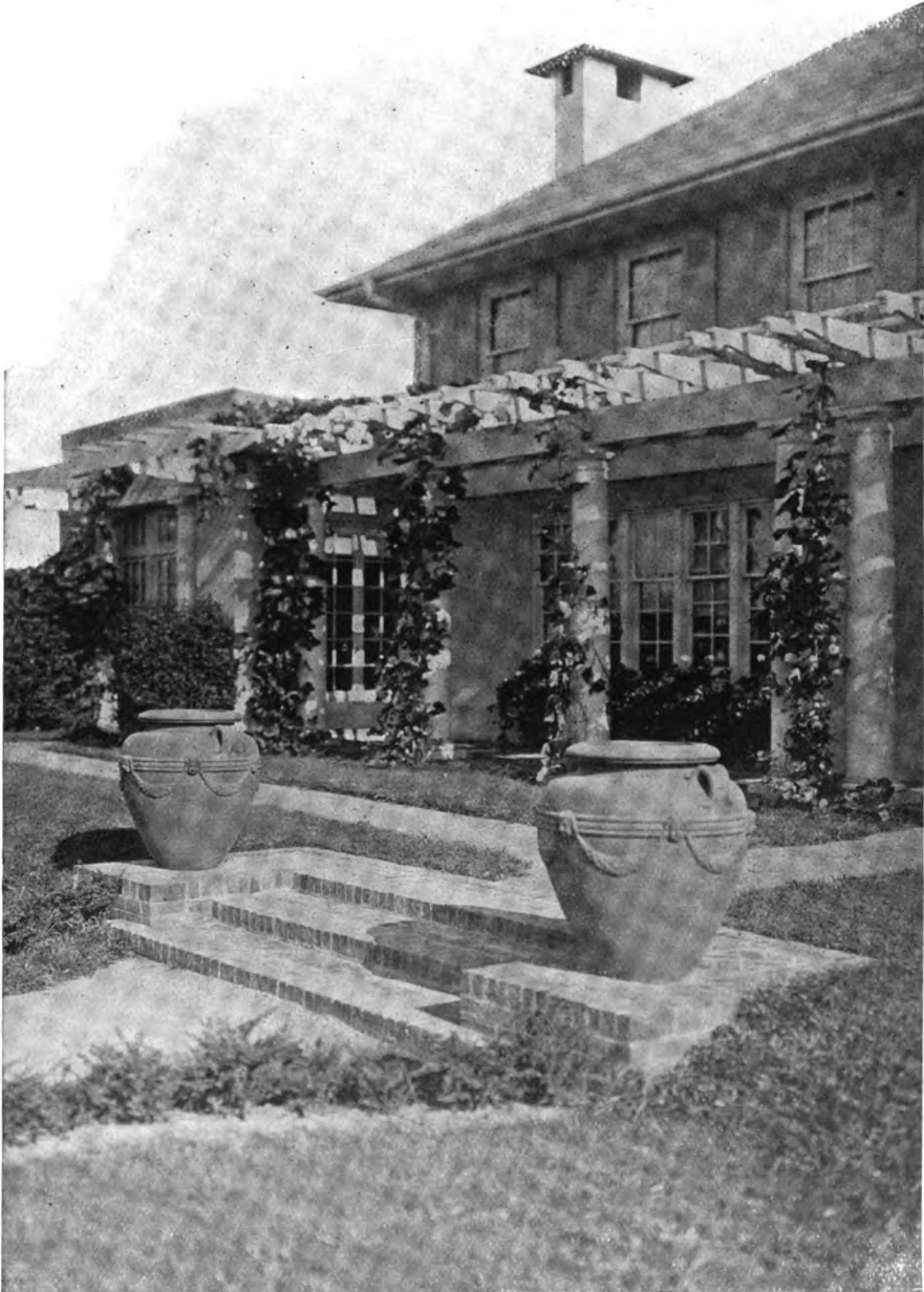
PERGOLA-PORCH FOR A COUNTRY HOUSE AT EAST HAMPTON, LONG ISLAND: THE PERGOLA PORCH IS RAPIDLY TAKING THE PLACE OF THE OLD-TIME PIAZZA.
